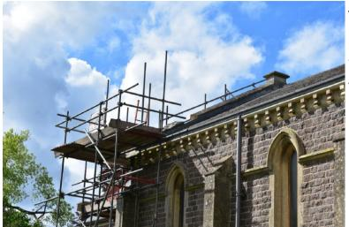
The stone coping on the gable end at the chancel end is delaminating which means that pieces are falling off.
