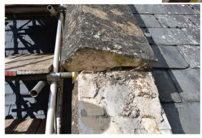
This resulted in water creeping back under the coping causing it to become saturated and prone to damage by frost. Roots of plants have been seen under the coping, having followed the water.
